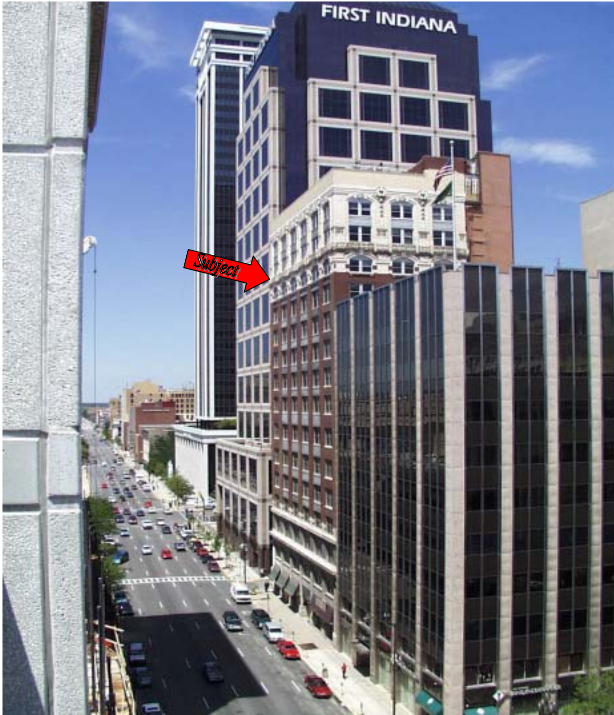
VIEW LOOKING NORTH ON PENNSYLVANIA
